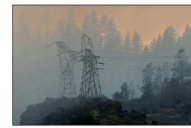
High voltage towers cling to the steep canyons around Pulga on Nov. 9, 2018, near the reported start of the Camp Fire blaze that destroyed Paradise and killed at least 85 people.
